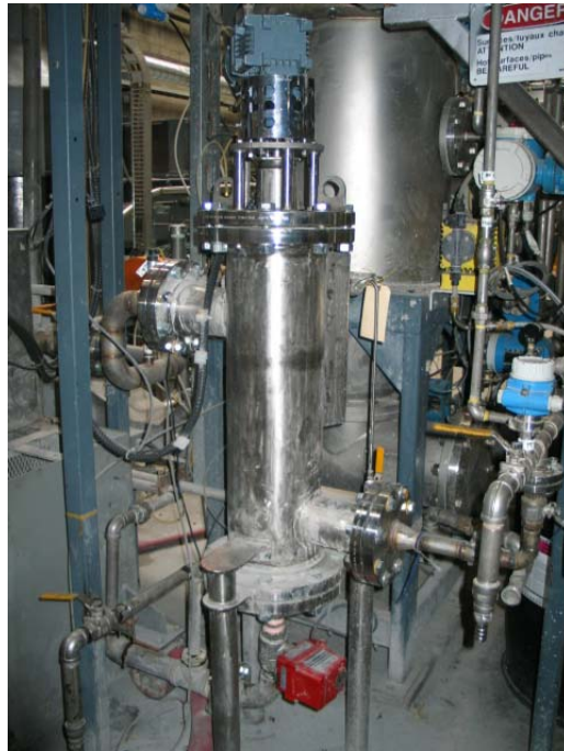
Figure 8 – New Self Cleaning Strainer
