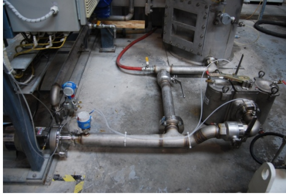
Figure 6 – New Pump & Suction Strainer Installation
